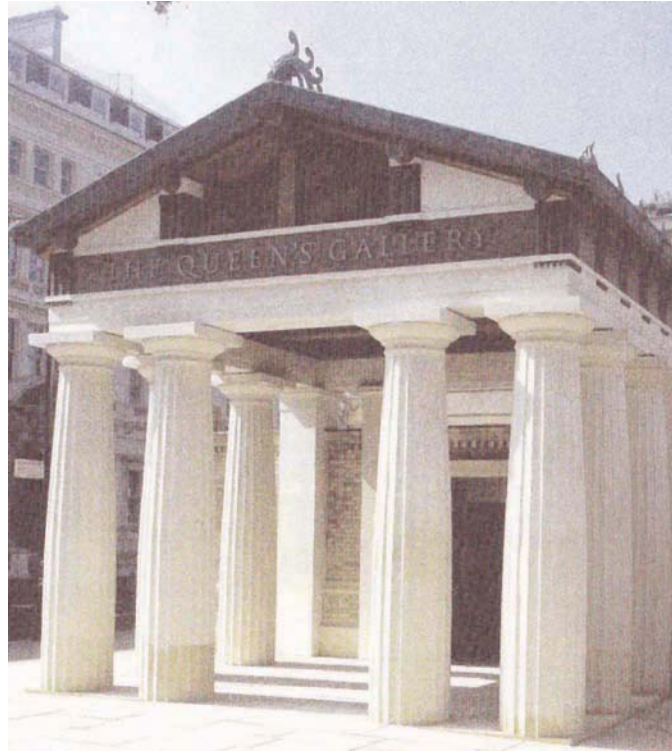
Fig. 10. The Queen's Gallery, Londyn, Wielka Brytania, arch. John Simpson, 2004r. New Civic Architecture The Ecological Alternative to Sub-Urbanization, Alinea, Firenze 2004
