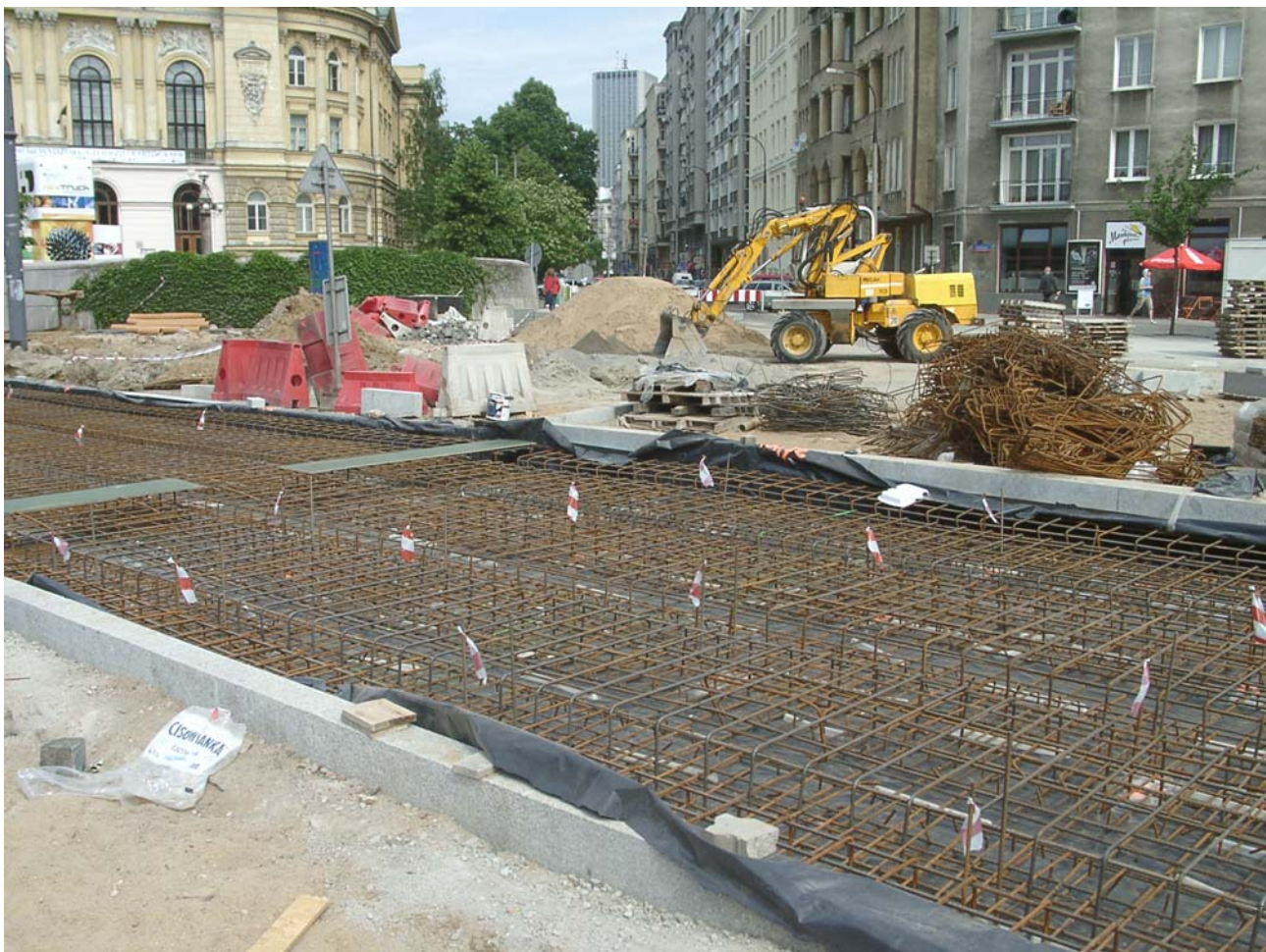
Fig. 9. The newest road construction technologies
