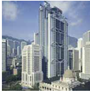
Fig. 3. Hongkong and Shanghai Bank in China ( http://www.architecturepics.org )
